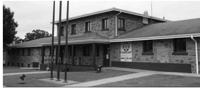
The St. Francois County Jail, completed in October 1996.
